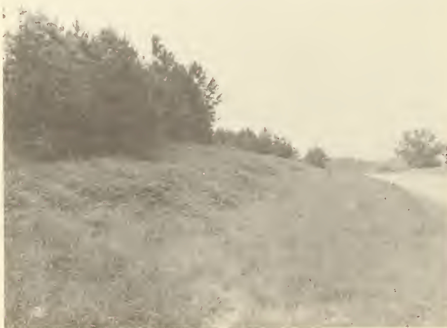
Figure 17.--A cover of honeysuckle that developed from natural stands is smothering out bahiagrass plantings on a roadbank of moderate slope. Honeysuckle, a vine plant, is useful on steep rough areas.
